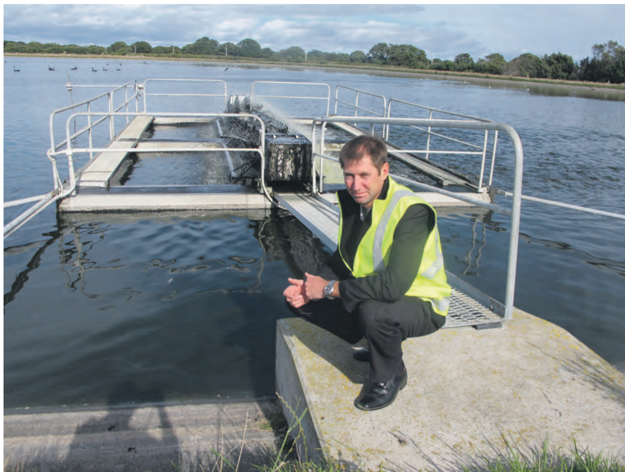
STDC group manager of engineering services in front of the Hawera waste water treatment plant.
